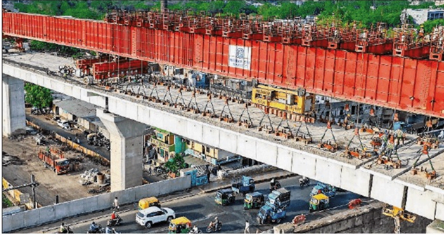
The structure rises about 19.5m from ground to rail level
